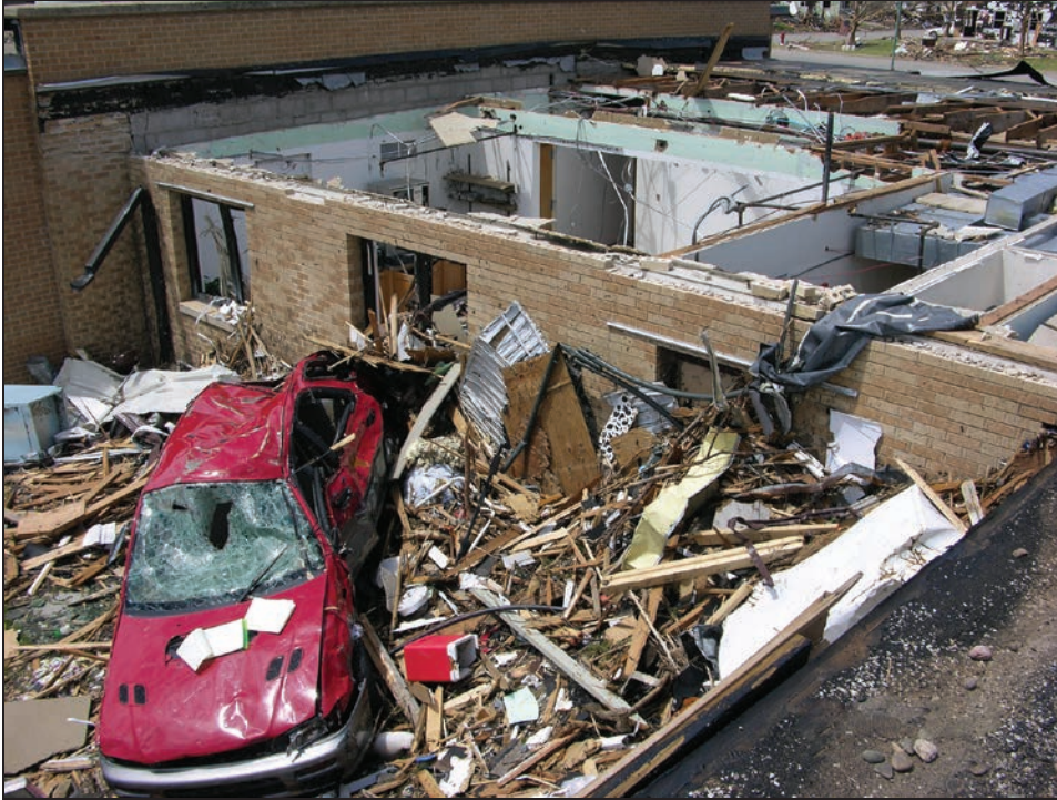
Figure B8-8. Representative quantity, size, and type of debris that is often generated by a strong or violent tornado. The building damage at this site was indicative of an EF3 tornado. (Greensburg, KS, 2007)
