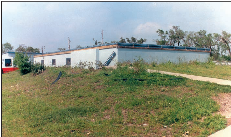
Figure B3-10. View of a community shelter that is partially below grade (Wichita, KS, 1999 tornado)
