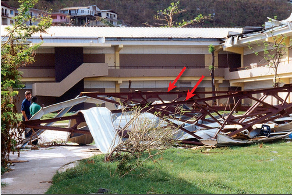
Figure B8-4. Large debris: Steel roof trusses that blew off a school (U.S. Virgin Islands, 1995 Hurricane Marilyn)
