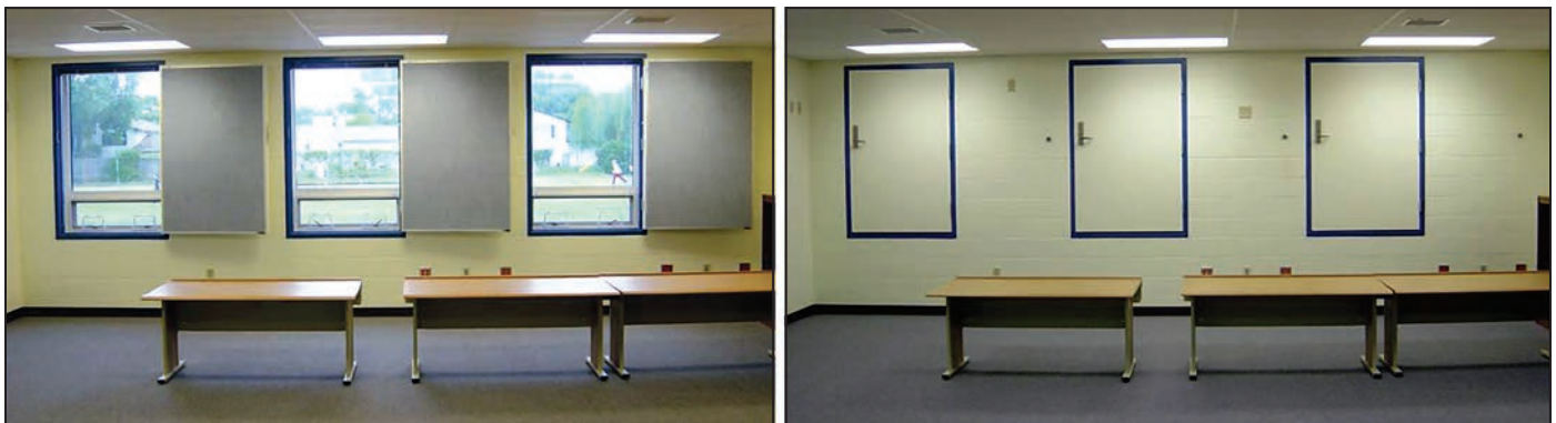
Figure A4-5. Interior-operated safe room shutters in a multi-purpose classroom/safe room. Image on left is normal usage; image on right shows shutters in “lock down” position where they are closed and latched
